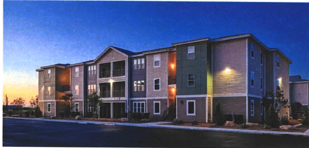
Wellspring | 144 Units | Pecos, TX | HUD Project No. 113-35793, National Green Building Bronze Certification
