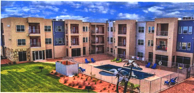
Eighty-Seventh | 181 Units | Odessa, TX | HUD Project No. 113-35686
